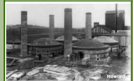
Former Brick Refractory in Howard, PA
